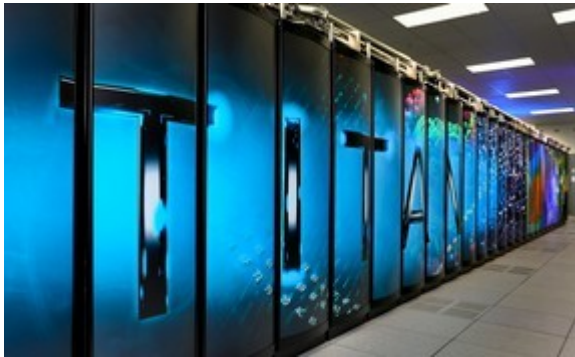
The Titan supercomputer has 18,688 GPUs
